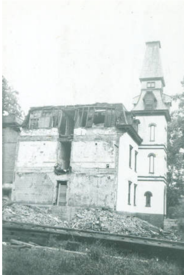
Demolition of Hartwick Seminary, 1946
